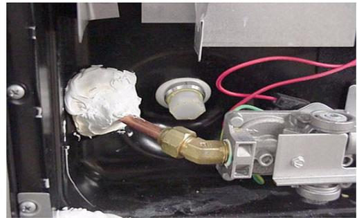
Also open the Pressure-Temperature relief valve at the top right portion of the tank to prevent air locking in the tank while draining.
