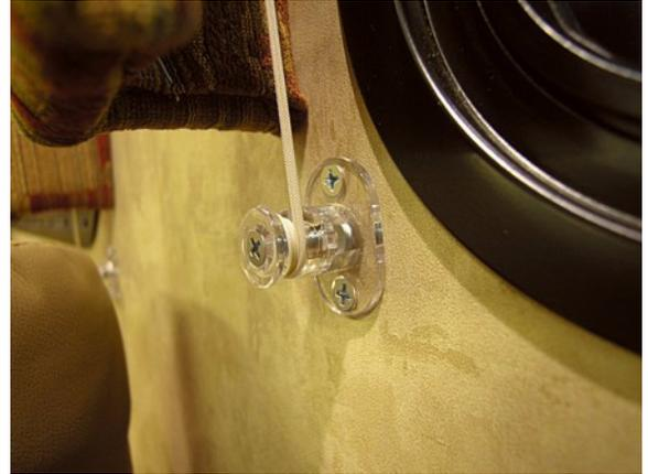
*To loosen the tension*, unwrap the guide cords from the spools one turn at a time until desired tension is achieved.
