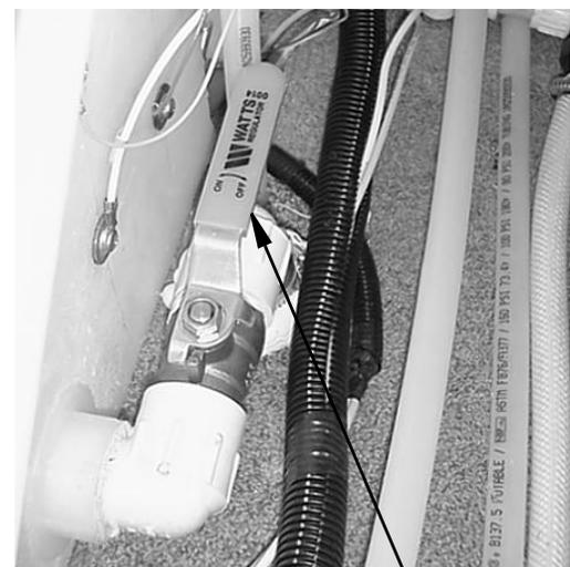
Water Tank Drain Valve
