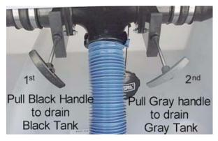
Holding Tank Dump Valves (Typical)
