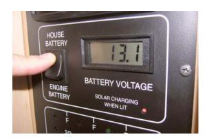
The LCD display will show the current battery voltage to the nearest tenth of a volt.
