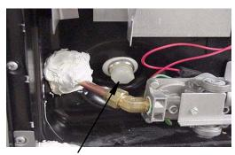
Water Heater Drain Plug (Remove with socket)
