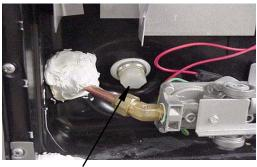
Water Heater Drain Plug (Remove with socket)
