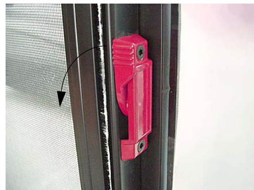
Pull latch outward to slide window open
