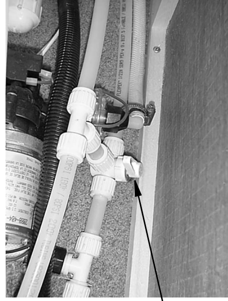
Water Line Drain Valve (Typical)
