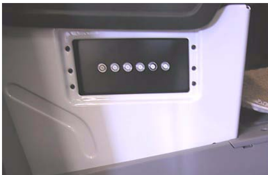
Chassis and House 12V Breakers on side of passenger seat base toward door (shown w/cover off)
