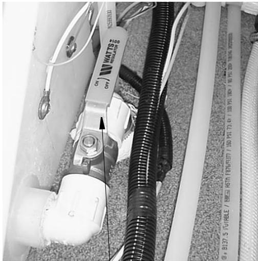
Water Tank Drain Valve (Typical)
