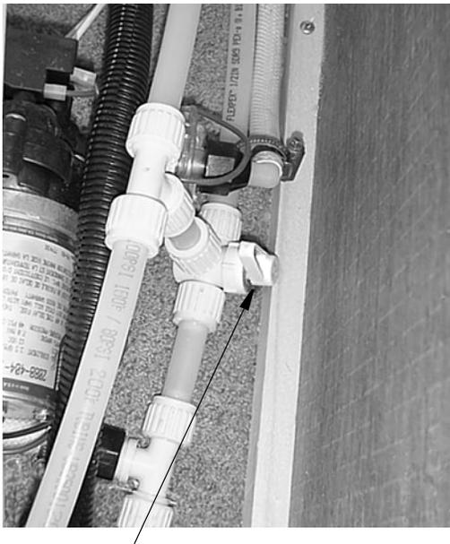
Water Heater Bypass Valve (Typical)
