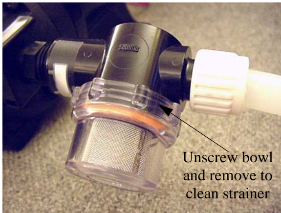
Water Pump Strainer (Located in water service center) -Typical View
