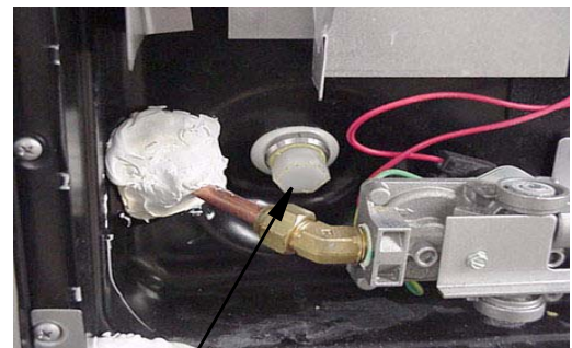
Water Heater Drain Plug Remove with socket.
