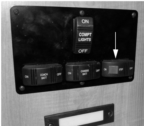
Entry Step Switch - Typical (Located near the entrance door)
