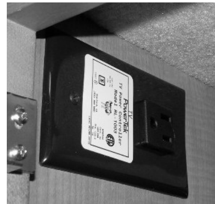
Front TV Ignition Switch Interlock -Typical View
