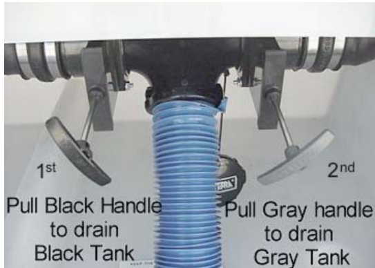
Holding Tank Dump Valves (Typical)
