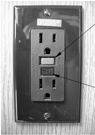
GFCI Outlet (Ground Fault Protector)
