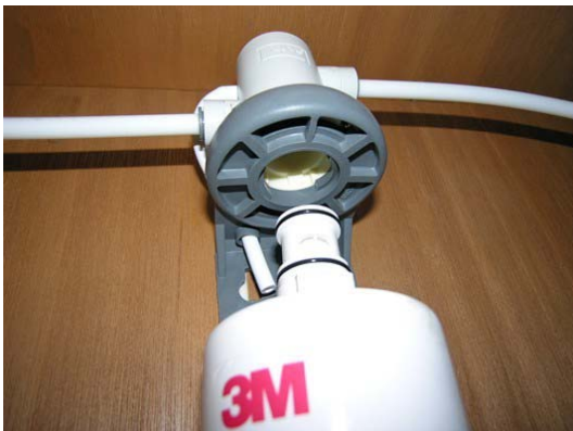
Insert new filter up into filter socket – Press and twist 1/4-turn clockwise
