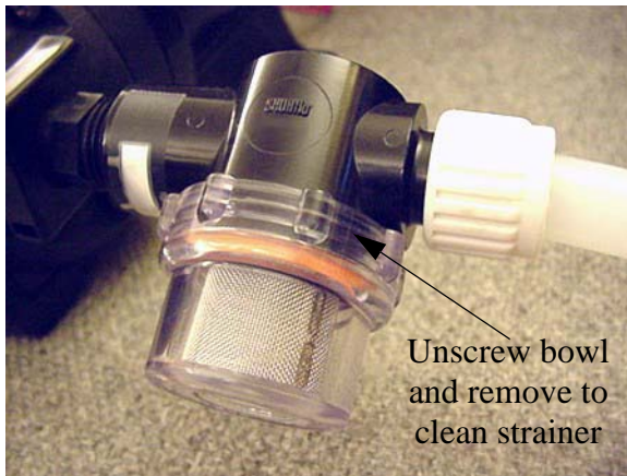
Water Pump Strainer -Typical View
