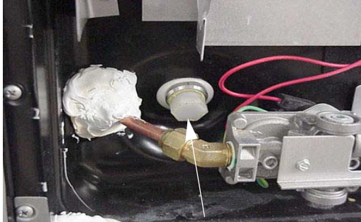
Water Heater Drain Plug (Remove with socket)
