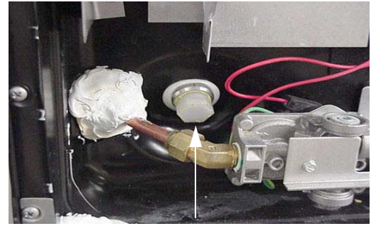
Water Heater Drain Plug (Remove with socket)
