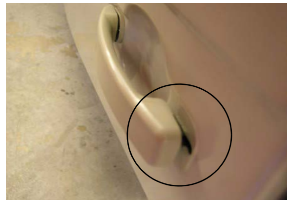
Door Unlatched (note gap)
