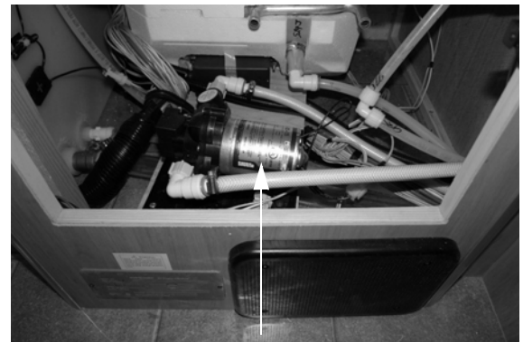
Water Pump (Located beneath wardrobe or refrigerator cabinet, depending on model) * Remove panel to access -Typical Installation
