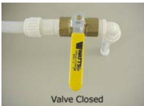
Water Tank Drain Valve (Typical)
