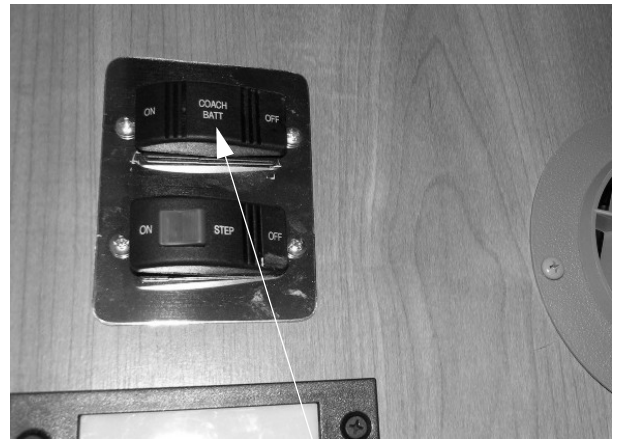
House/Coach Batt Disconnect Switch
