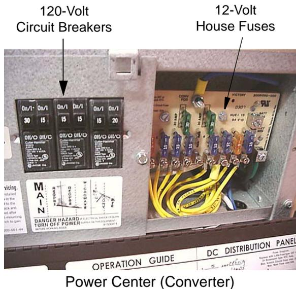
Certain circuits, however, remain unchanged for use by items which require 120-volt current, such as the air conditioner(s), the refrigerator in AC mode, the microwave oven, etc.
