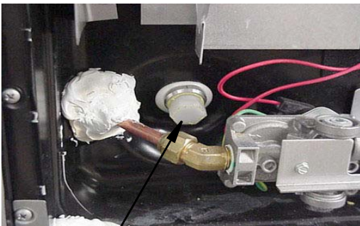
Water Heater Drain Plug (Remove with socket)
