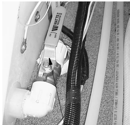
Water Tank Drain Valve (Typical)
