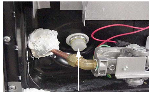
Water Heater Drain Plug (Remove with socket)
