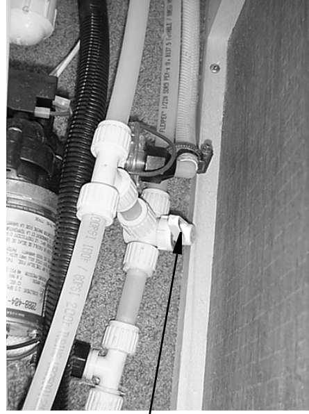
Waterline Drain Valve (Typical)
