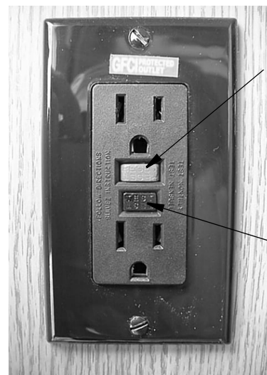
GFCI Outlet (Ground Fault Protector)
