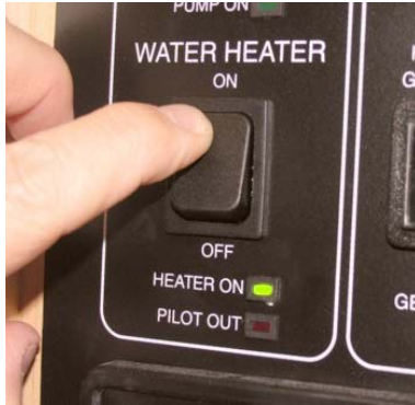
Gas Water Heater Switch (Located on Systems Monitor Panel)
