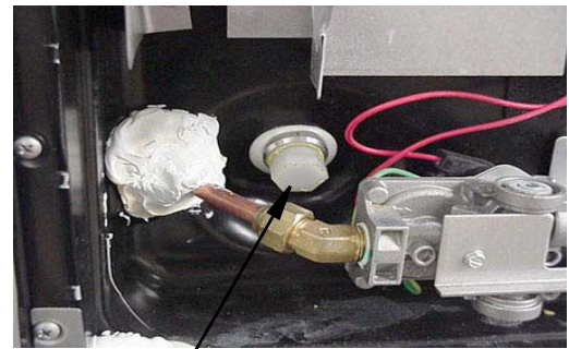
Water Heater Drain Plug (Remove with socket)
