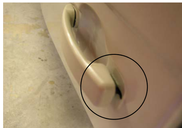
Door Unlatched (note gap)
