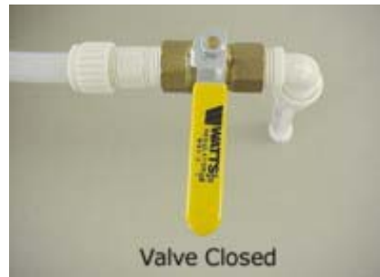
Water Tank Drain Valve -Typical installation shown
