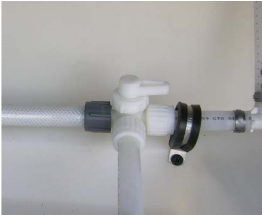
Waterline Drain Valve -Typical installation shown
