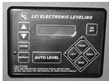
Leveling System Control Panel (Located on dash)
