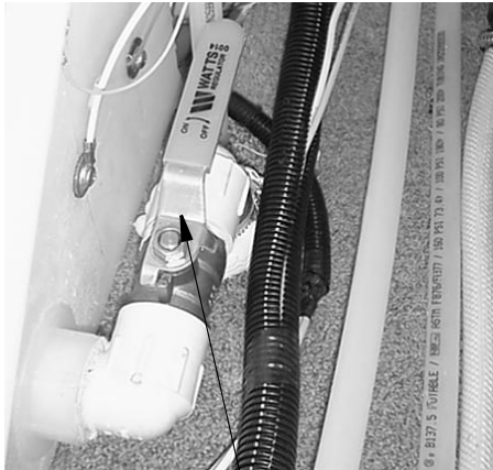
Water Tank Drain Valve (Typical)
