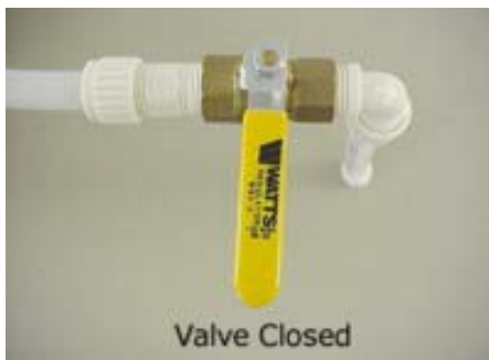
Water Tank Drain Valve (Typical)
