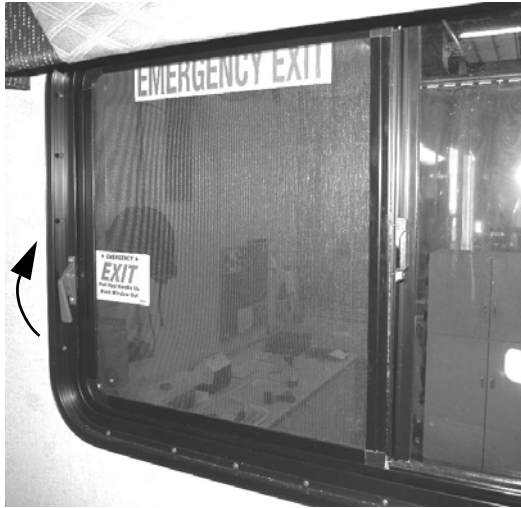
Bedroom Escape Window (Lift both red safety latches UP and push window OUT for emergency exit) -Typical View
