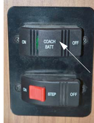
House/Coach Battery Disconnect Switch (Located near entrance door or end of galley, depending on model) -Typical View
