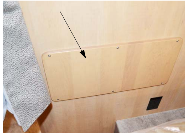
Refrigerator Access Panel (Located on front bedroom wall) *Model 23T
