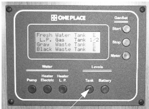
Tank Levels Switch
