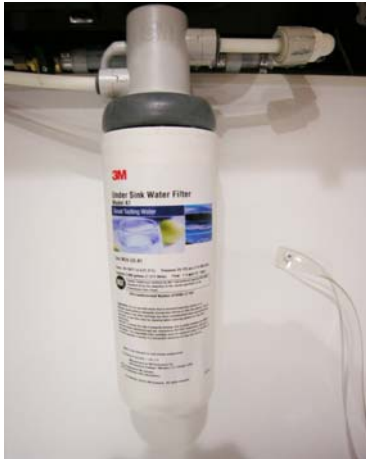
Galley Cold Water Faucet/ Ice Maker Filter Assembly (Located below galley sink) -Typical View
