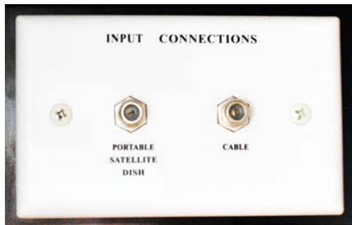
Satellite Dish and Cable TV Connections (Located in utility compartment, shoreline compartment, or water service center, depending on model) -Typical View
