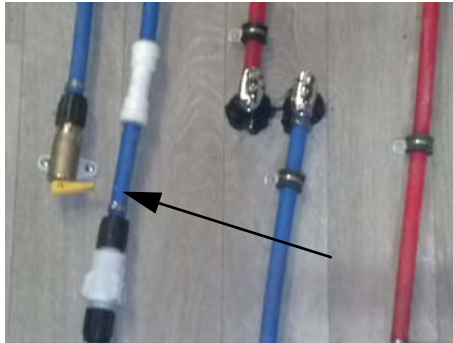
Pressure Relief/Drain Valve (Yellow) (See “Water System Drain Valve Locations” chart at the end of this section for location on your model)
