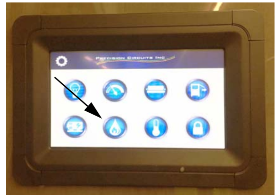
Water Pump Switch
