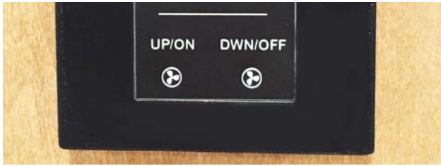
Power Roof Ventilator Switches
