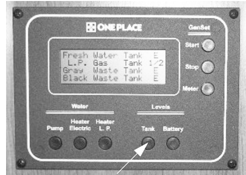
Tank Levels Switch
