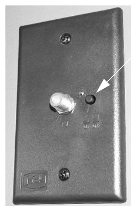
TV Signal Amplifier Power Switch (Located in an overhead cabinet or mounted on a wall near the TV) -Typical View
