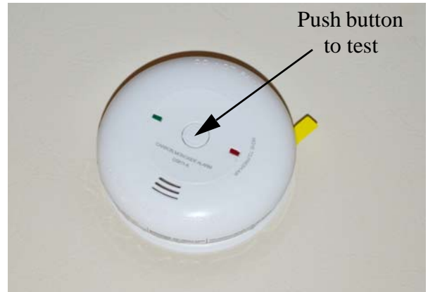
Carbon Monoxide Alarm
