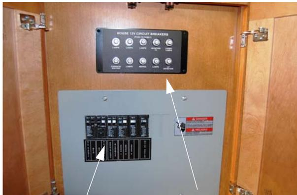
120-Volt House Circuit Breakers      12-Volt House Circuit Breakers
