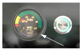
Pure<sup>3</sup> State of Charge (SOC) Gauge (Located on an interior cabinet)
