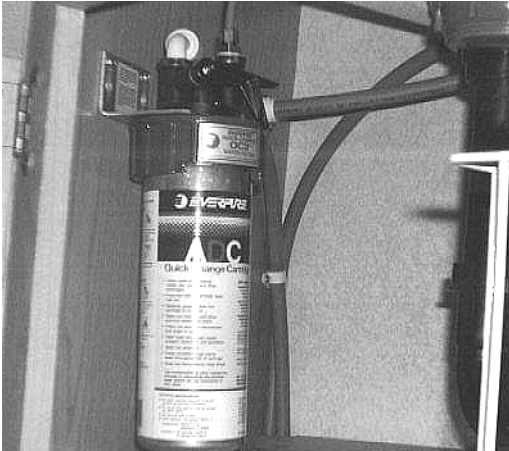
Water Filter Assembly - Below Galley Sink
