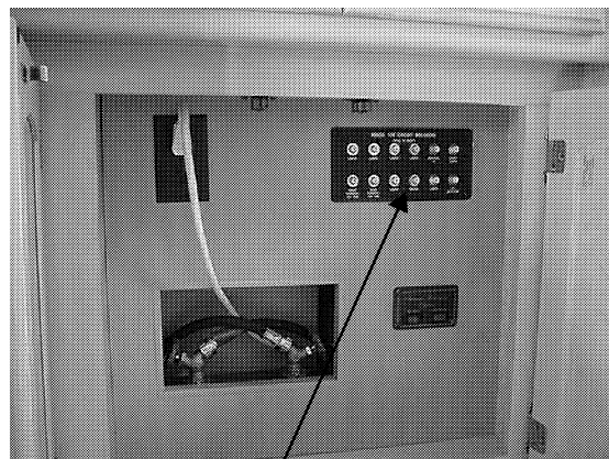
House 12V Breakers Model 40J
