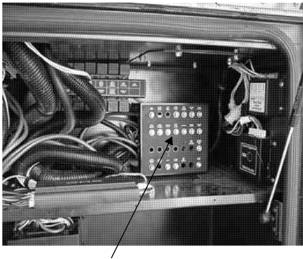
Automotive 12-Volt Breaker Panel
