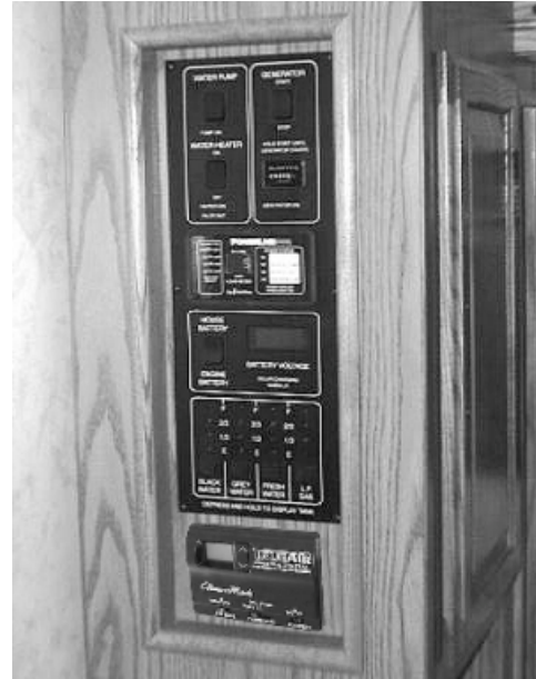
One Place Monitor Panel
