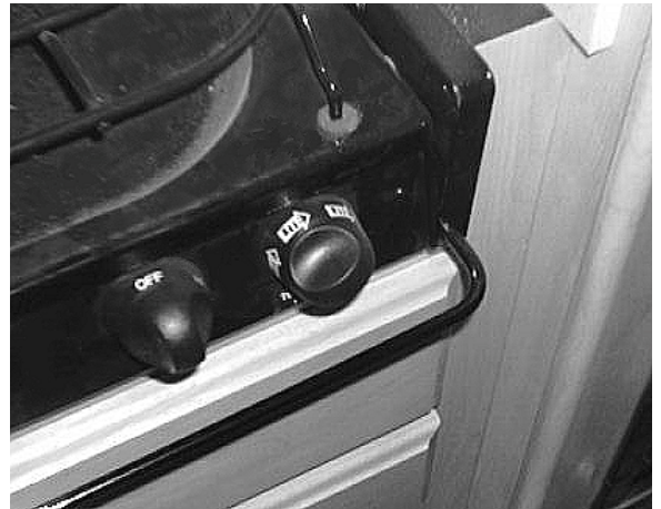
Rotate knob in direction of arrow while turning burner on to light
