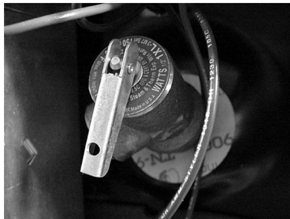
Lift straight out to open P-T valve
