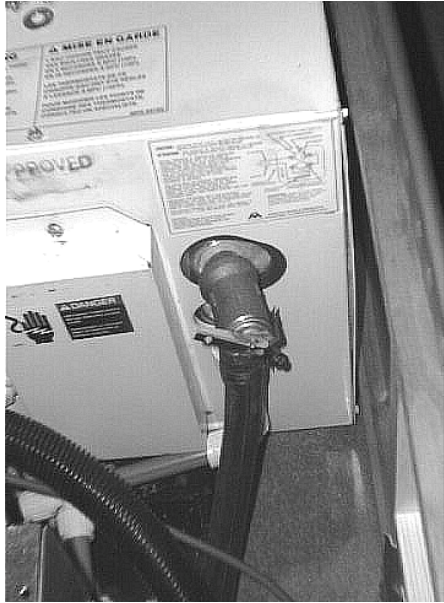
Pressure-Temperature Relief (P-T) Valve
