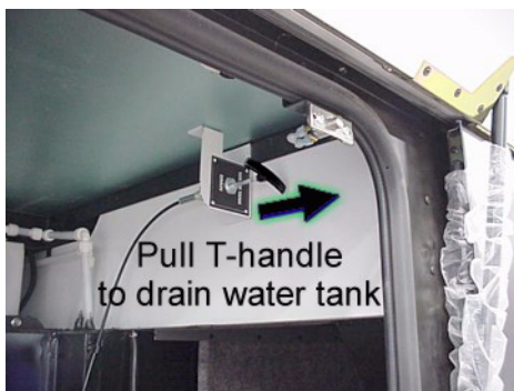
Water Tank Drain
