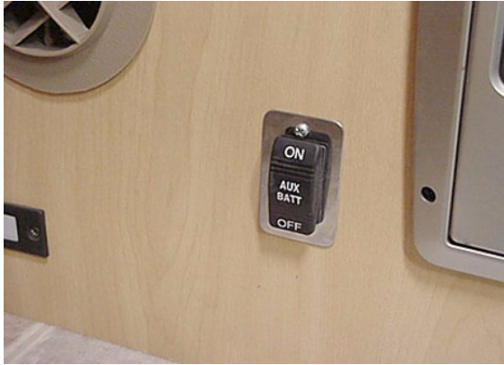
Aux. Batt. Switch (Near entrance door)
