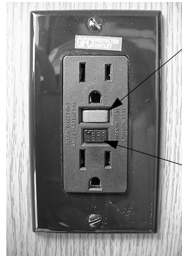
GFCI Outlet (Ground Fault Protector)
