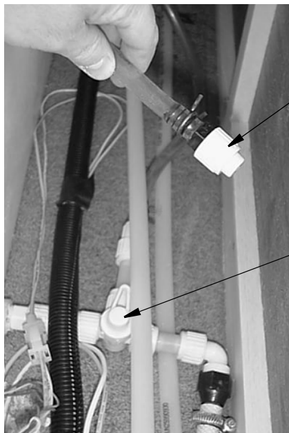
Winterization Valve (See chart at end of section for location)
