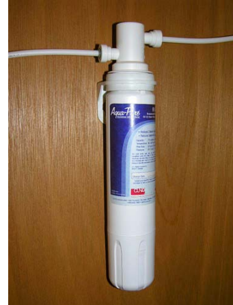
Water Filter Assembly (Located below Galley Sink) * Typical View - your coach may vary
