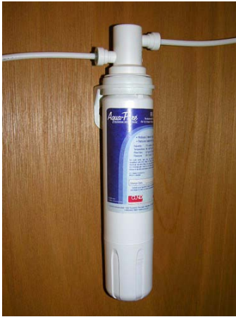
Water Filter Assembly (Located below galley sink)
