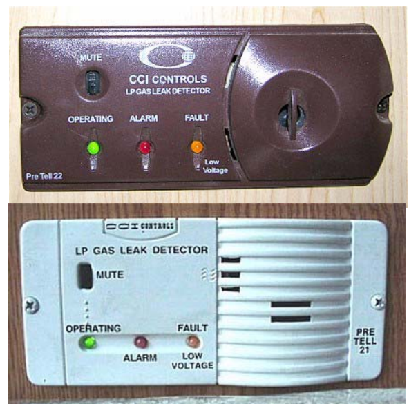
Propane Gas Leak Detectors (typical)
