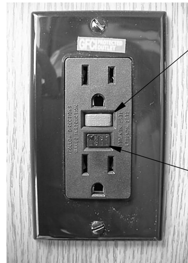
GFCI Outlet (Ground Fault Protector)
