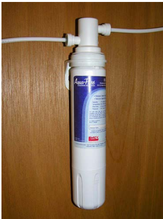
Water Filter Assembly (Located below galley sink)
