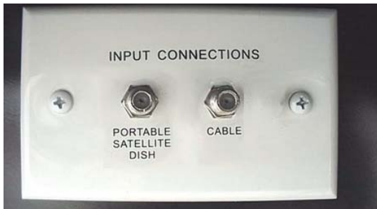
Satellite Dish and Cable TV Input (Hook-Up) Connections (in Utility Compartment)
