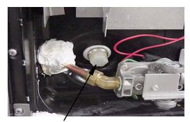
Water Heater Drain Plug Remove with socket.
