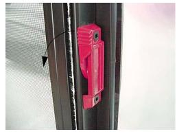
Pull latch outward to slide window open
