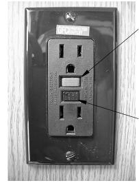
Push to Reset circuit after monthly testing or ground fault tripping.
