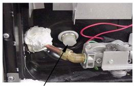
Water Heater Drain Plug Remove with socket.
