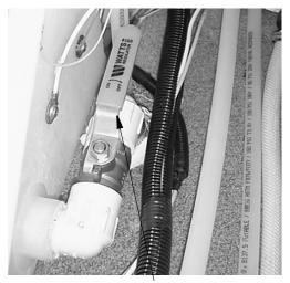
Water Tank Drain Valve (Typical)
