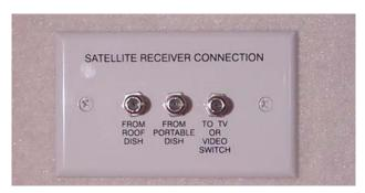
Interior Connection for Satellite Dishes (in overhead cabinet near TV\*)
