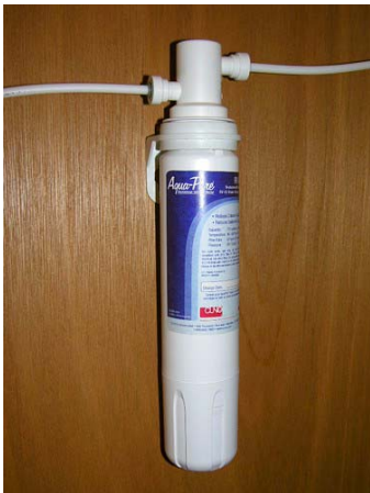
Water Filter Assembly below Galley Sink
