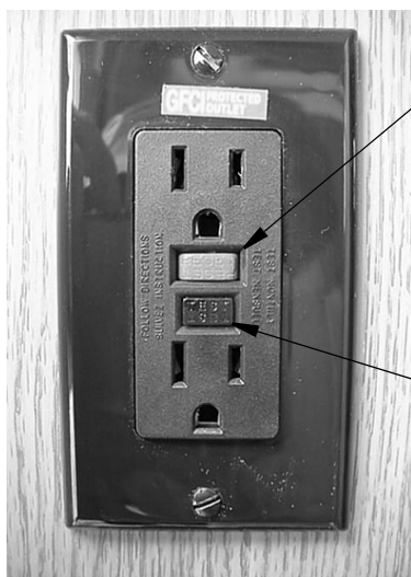
GFCI Outlet (Ground Fault Protector)
