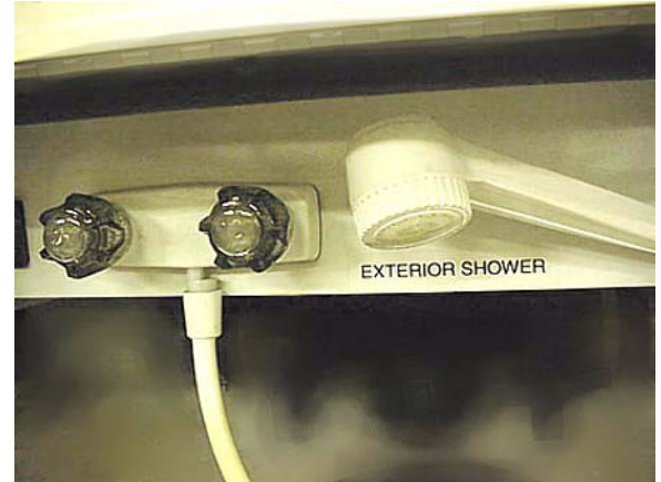
Exterior Shower/Wash Station (typical)
